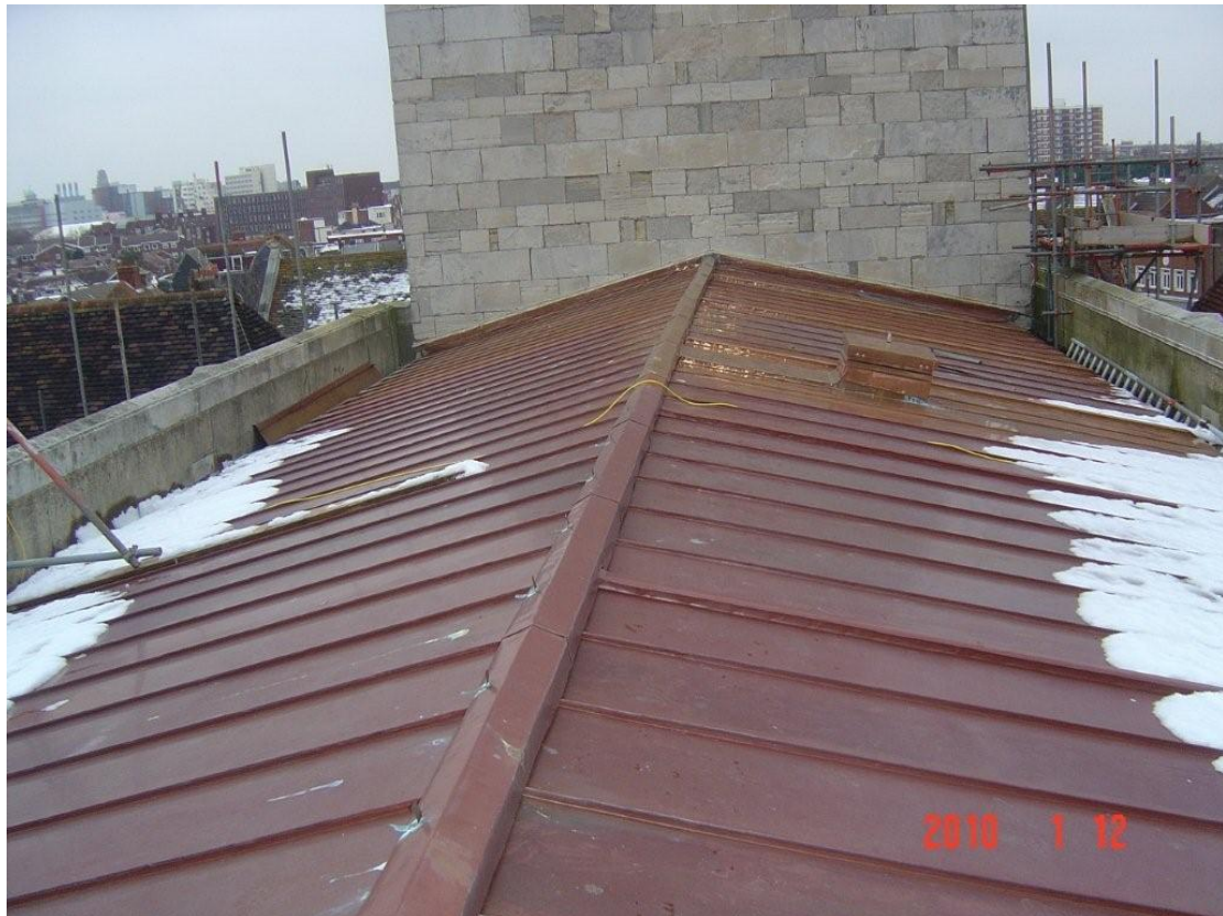
New copper roof over the Nave main aisle
