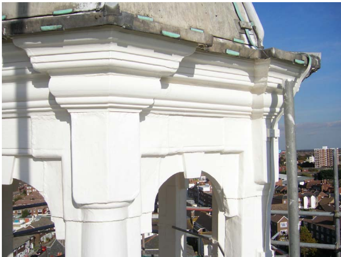
Repaired and redecorated lantern – south facing elevations.
