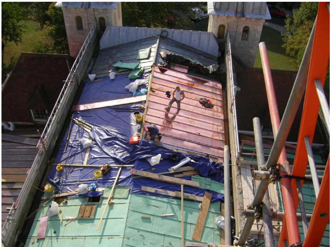
Long strip copper roofing to Nave roof – north slope.
