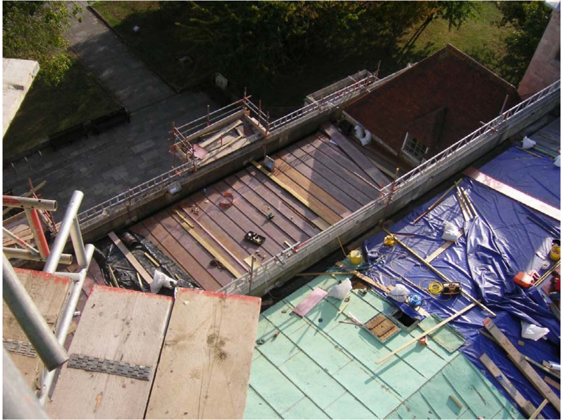
Long strip copper roofing to South Aisle roof.
