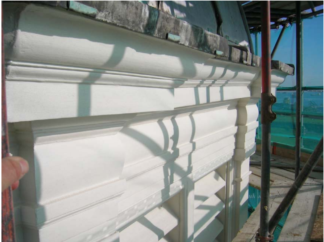
Cornice and mouldings above Octagon Louvres to the Belfry.
